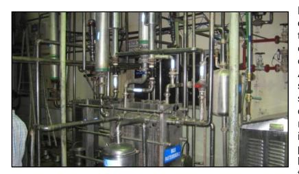
Bhopal dairy plant is the first dairy in the Madhya Pradesh to be computerized with the existina facility and equipments. Dairy Automation Pvt. Ltd. has successfully introduced full scale automation of all critical process like Milk reception, Chilling, Storage in raw milk silos, operation of pasteurizer. separator, homogenizer, milk dispatch Packing section
